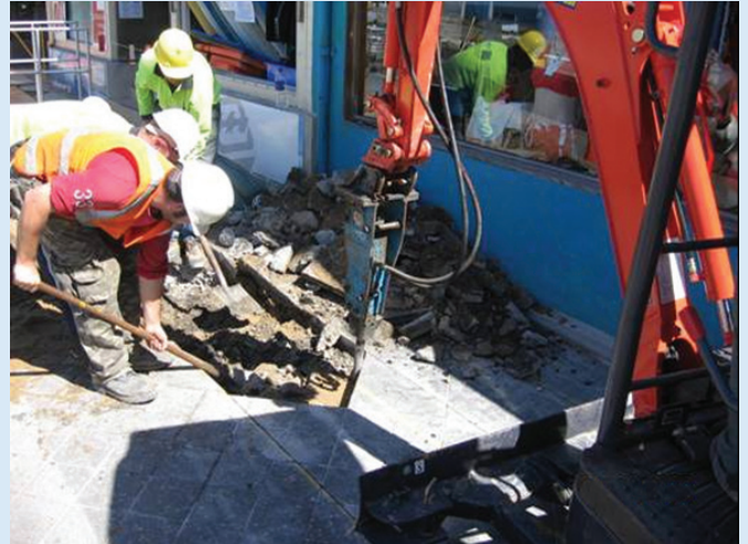
Trenching work similar to that being undertaking in King Street, Newtown.
