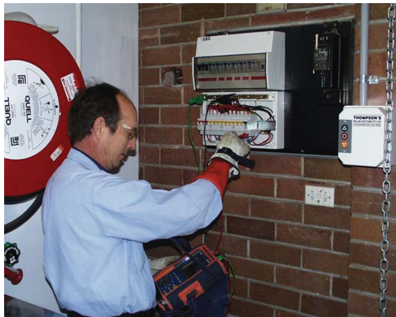
Figure 1 - Installation inspector tests a distribution sub board
