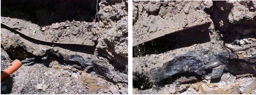
Bitumen encased cable with Polymeric Cable Cover
