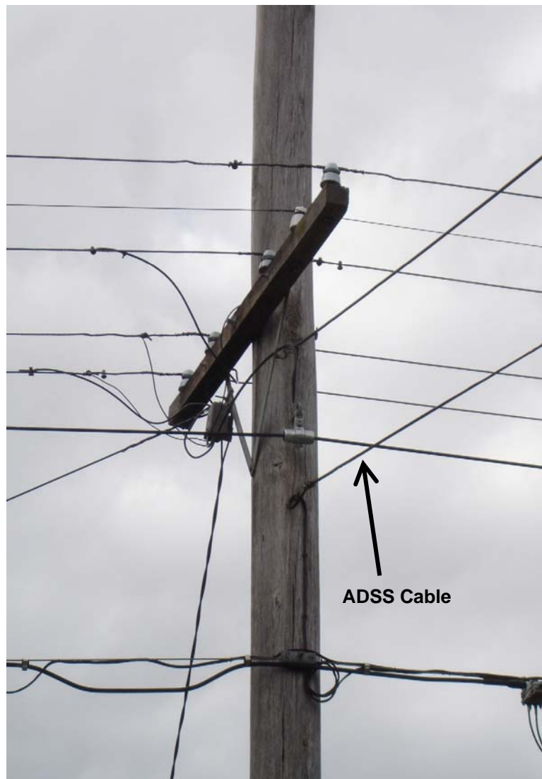
Figure 6: Typical ADSS installation
