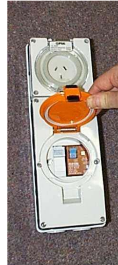
Figure 8: Consumer terminal box with optional GPO
