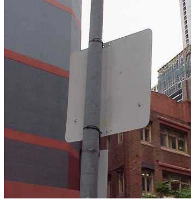
Figure 22: Sign inappropriately secured using plastic cable ties
