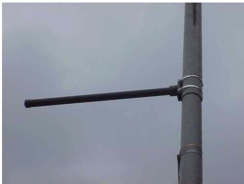
Figure 23: Banner support arm secured with approved stainless steel band clamps
