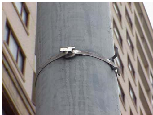
Figure 24: Banner base anchor secured with approved stainless steel band clamps
