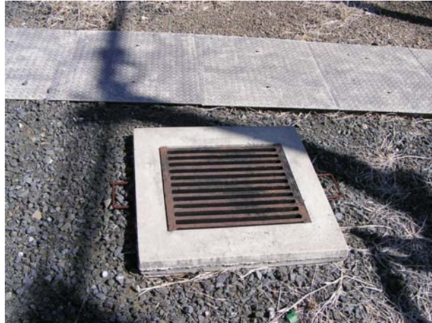
Figure 3: Typical Stormwater Pit
