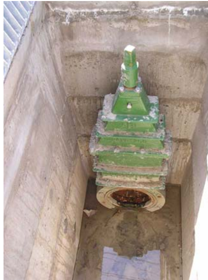
Figure 10: Knife Gate Valve
