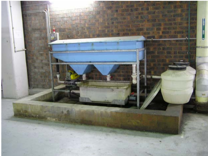
Figure 11: Typical Plate Separator
