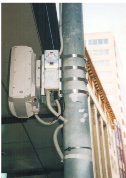
Figure 1 Microcell installation
