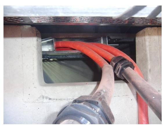
Figure 13 – New cutout section between the transformer oil compartment and the HV section for the transformer cables
