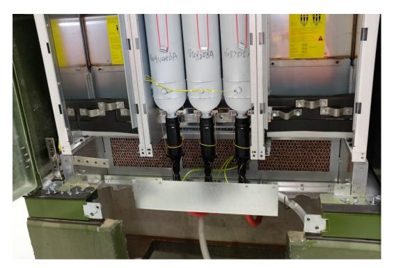
Figure 16 – Cable installation with full access
