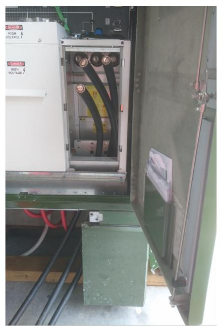
Figure 14 – Cable installation with limited access
