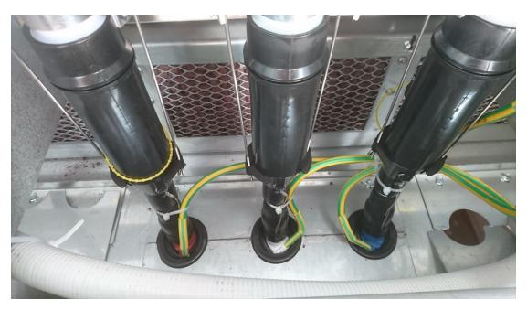
Figure 11 – Transformer cables in tee-off endbox
