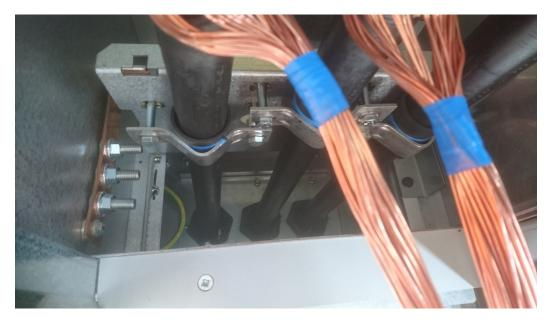
Figure 9 – Cable entry into RHS endbox (early version of cleat bracket and earth bar)
