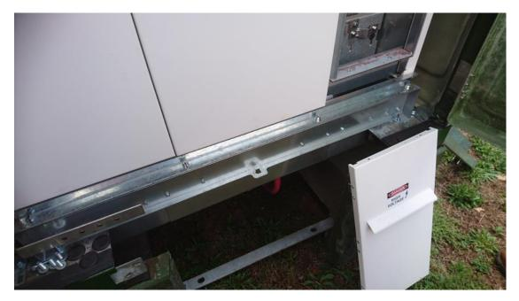
Figure 7 – Top lintel (Fibreglass), D-pull handle lintel, Concrete base access cover (lintel) and RHS endbox cover removed
