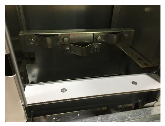
Figure 8 – Cable cleats and bracket inside RHS endbox
