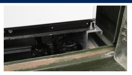
Figure 12 – Existing cable cleat bar now replaced by internal endbox bracket and supports
