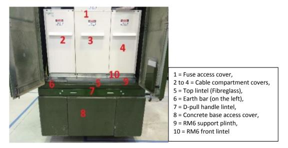
Figure 5 – New IAC KL type kiosk showing access components at the HV doors
