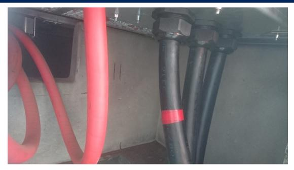
Figure 10 – Cable entry into bottom of RHS endbox
