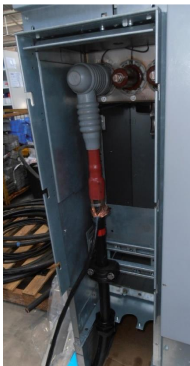
Figure 14 – Ring feeder endbox, showing cleat bar with split gland plate and front covers removed
