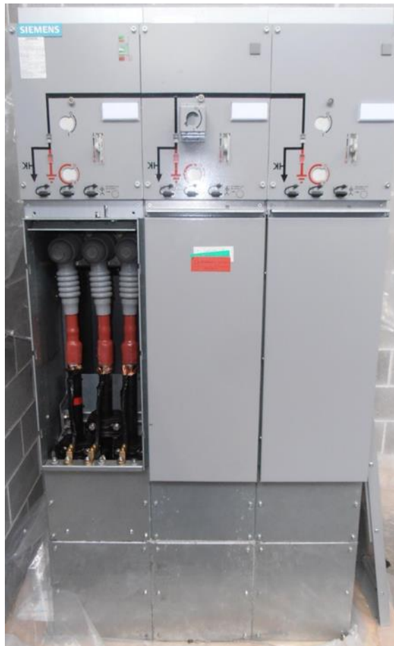
Figure 1 – 8DJH 'RRR' unit.
