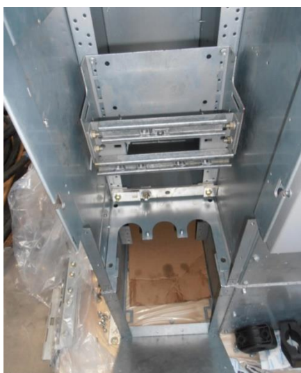
Figure 14 – Ring feeder endbox, showing cleat bar with split gland plate and front covers removed
