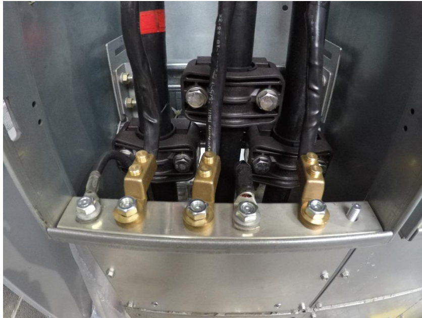
Figure 16 – Screen and earth connections, showing 2 off 70mm 2 cables connected to main earth bar.
