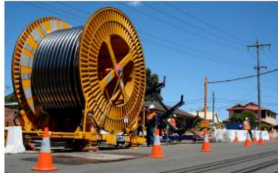
Cable installation on a similar project
