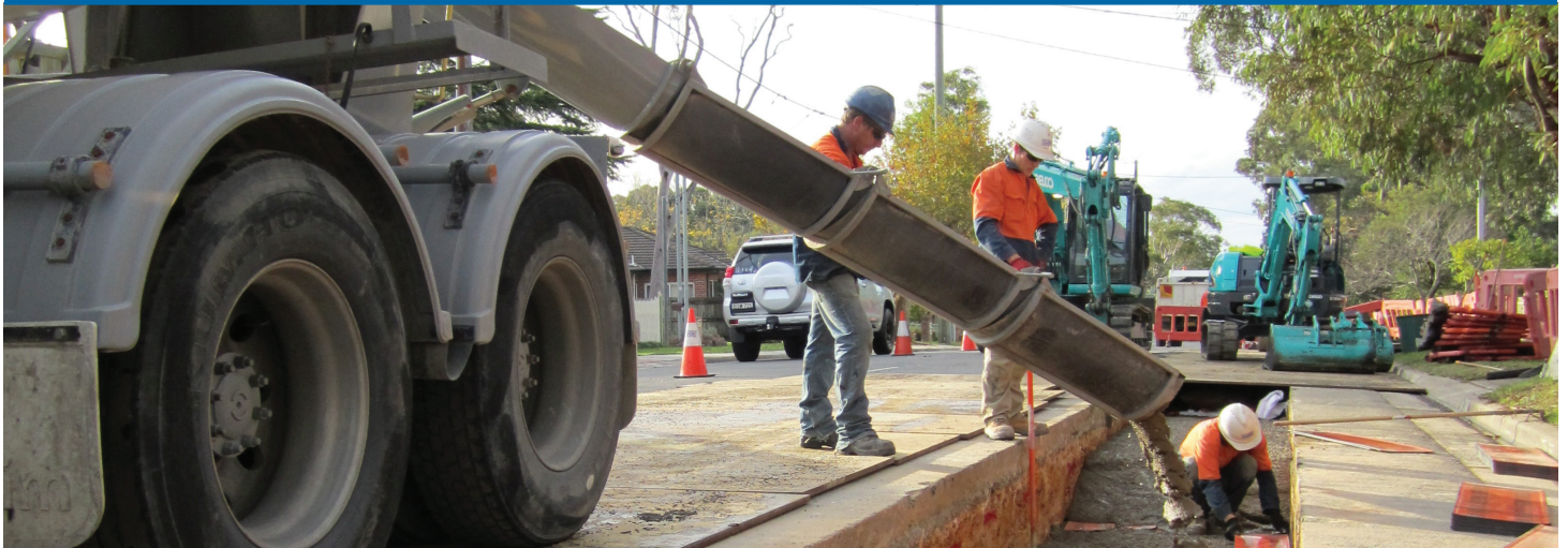
A similar cable project in progress
