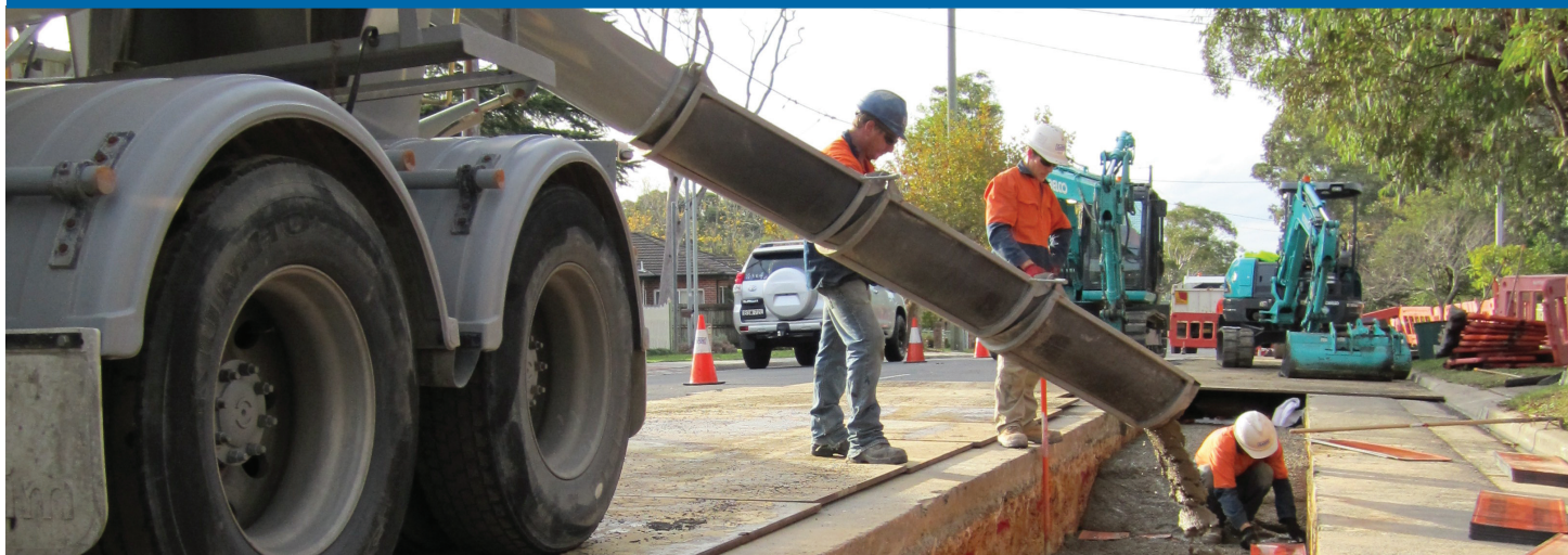
A similar cable project in progress
