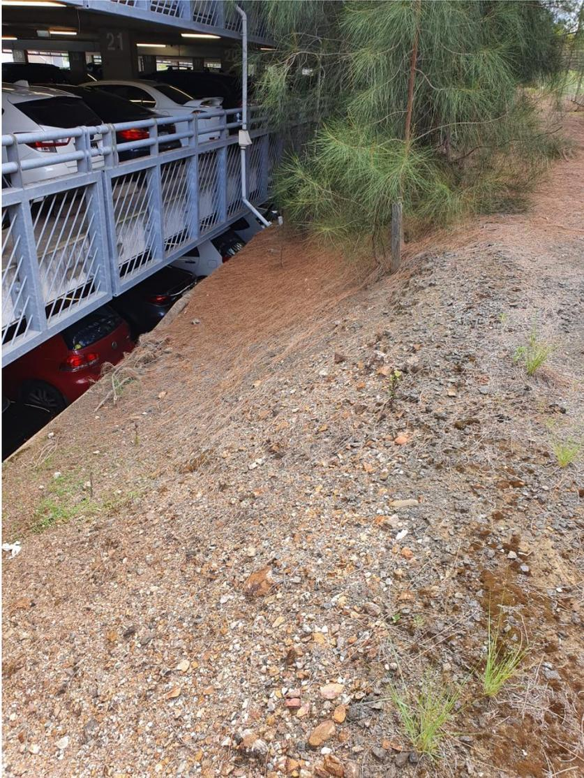
**Figure 5** - Image indicating the drop off from the raised level top of the berm and the steep sloping side-slope of the fill to the retaining wall about 1m below the crest.
