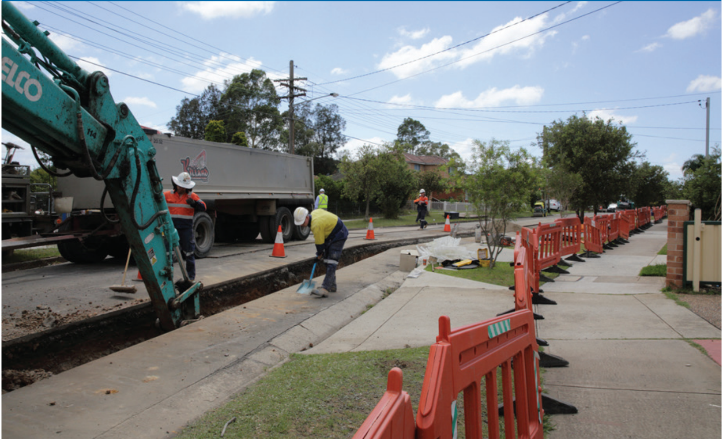
A similar cable project in progress
