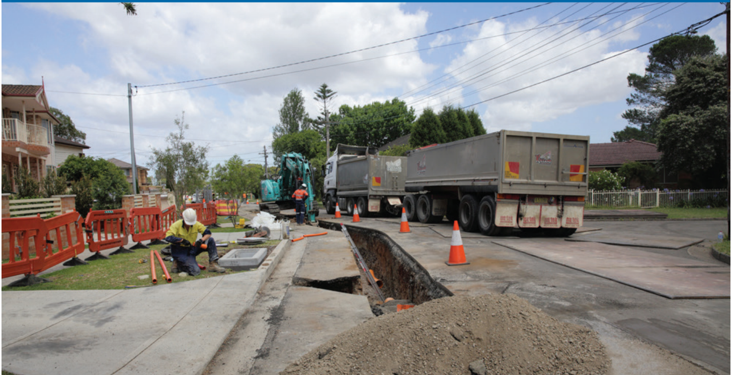
A similar cable project in progress
