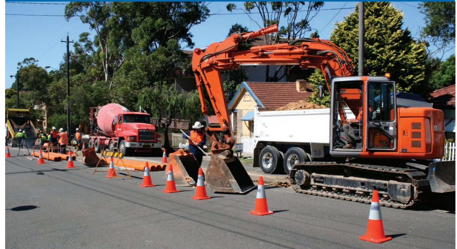
A similar cable project in progress
