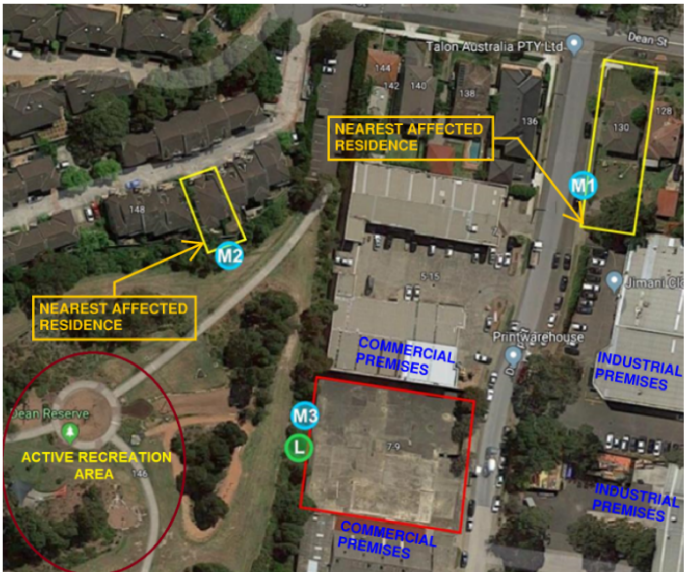
Figure 1 : Aerial view of site. The proposed development is outlined in red sharing boundaries with industrial premises to the north and south. The nearest affected residences are outlined in yellow and the Active Recreation Area circled in brown. Long term logger measurement location is marked as L in green and operator attended measurements M1-3 in blue.
