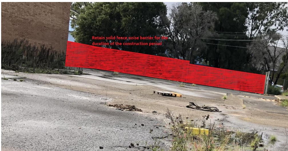
Figure 4: Recommended minimum noise barriers during construction. (north-east)
