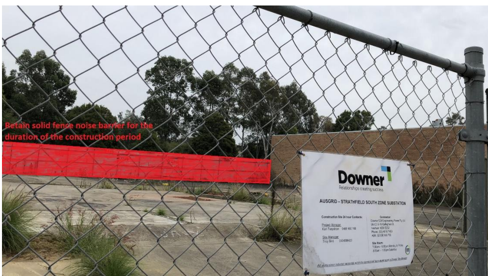
Figure 2: Recommended minimum noise barriers during construction.
