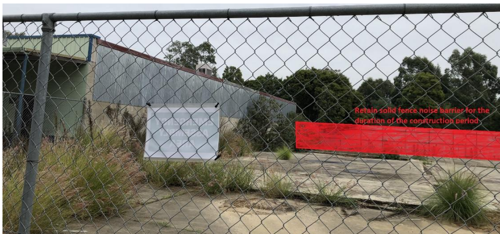
Figure 2: Recommended minimum noise barriers during construction. (south-west)
