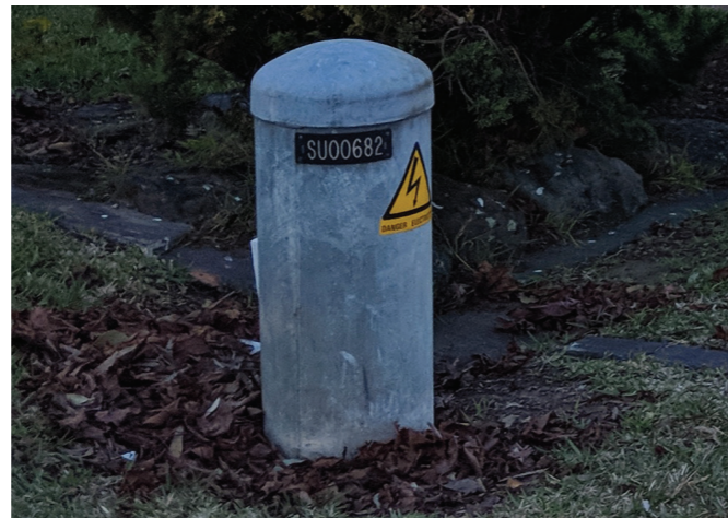
Typical pillar to be replaced
