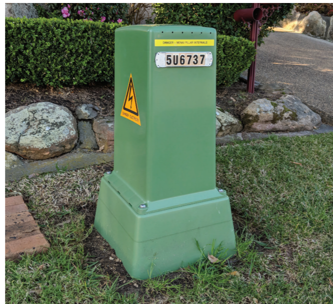
Typical current standard pillar to be installed
