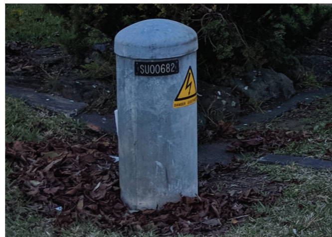
Typical pillar to be replaced
