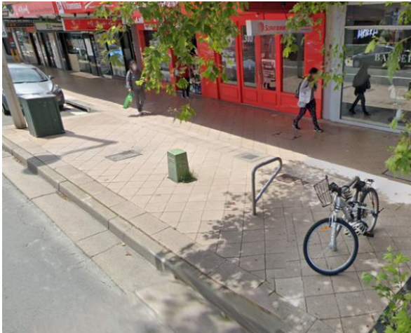
Fig B19 - Unacceptable – Low pillar in a commercial footpath and remote from other assets.
