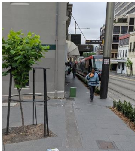
Fig B23 - Unacceptable – Low distribution pillar too close to building corner.
