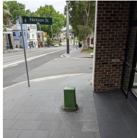
Fig B20 - Unacceptable – Near a doorway and middle of footpath with building setback.
