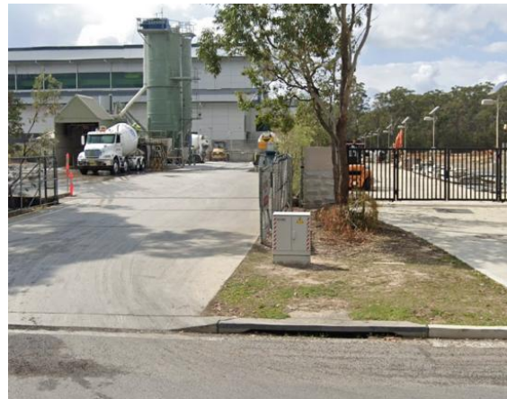
Fig B28 - Acceptable – Location meets the requirements but additional setback from driveway and/or bollards would reduce the risk of large vehicle impacts.
