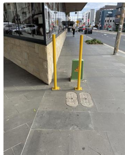
Fig B24 - Unacceptable – Low distribution pillar too close to building corner.
