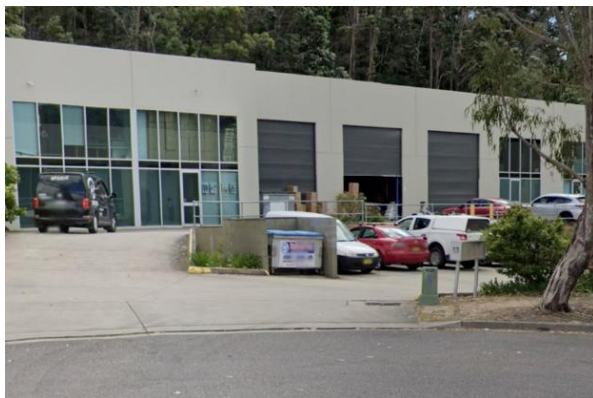
Fig B29 - Unacceptable – Low pillar with significant risk of vehicle impacts.
