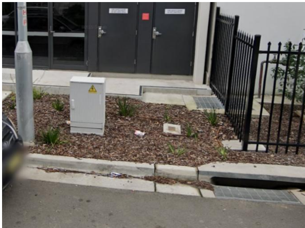
Fig B27 - Good – inside the property line and does not impede pedestrian access (future risk of garden overgrowth).
