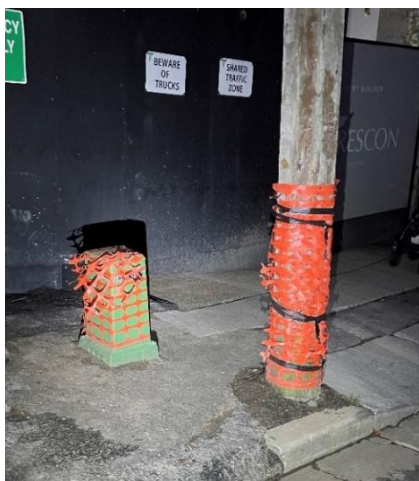
Fig B7 - Unacceptable – Low pillar is opposite existing pole and further impedes narrow footpath.
