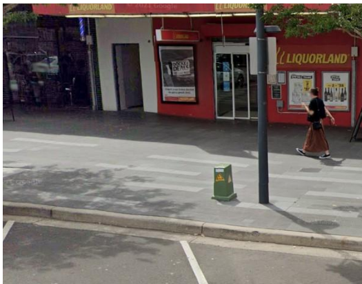
Fig B15 - Acceptable – Low pillar, but in line with other assets and within 1m.
