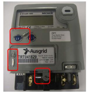
Figure 8.4-7 Seals that must remain intact
