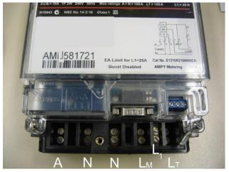
Figure 5.2-3 Wiring terminals of AMJ
