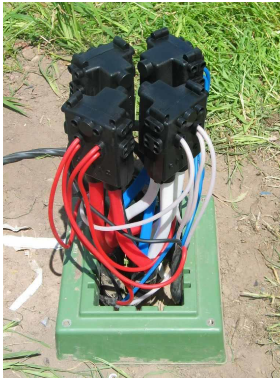
Figure 22.4 – Completed Three Way Pillar with turret removed
