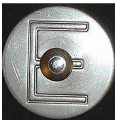
Figure 13: Approved kerb marking
